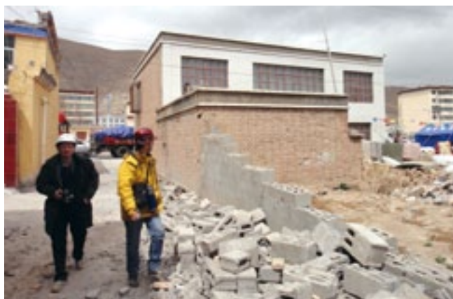
Tsinghua Experts Checking the Building Conditions in the Disaster Area
