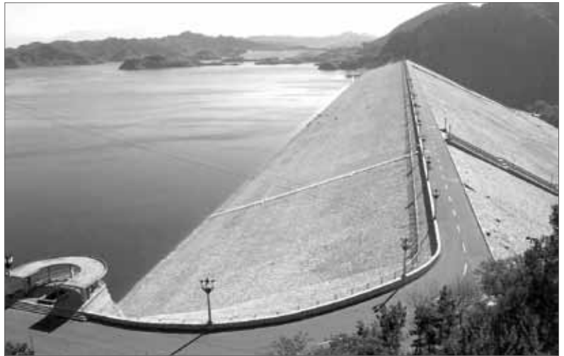
Reinforced Dam on the Chaobai River
